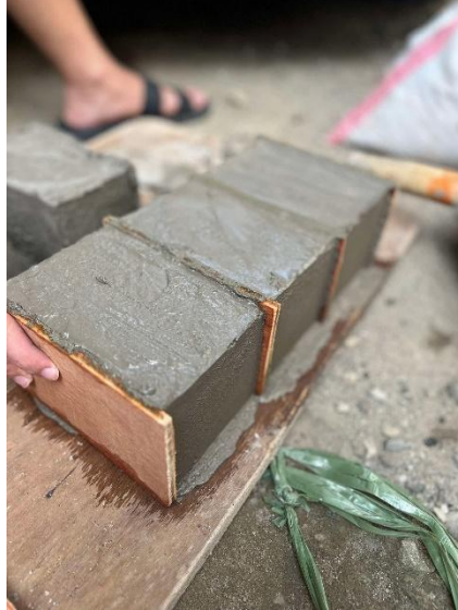
Removing the Molder
