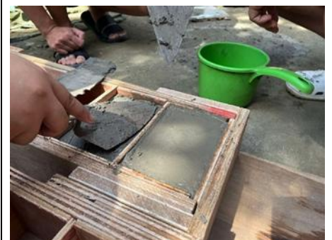
Leveling the Top of the Mold
